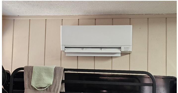
Below is the inside cassette for the Mitsubishi heat unit, 2 in each Cabin #6
